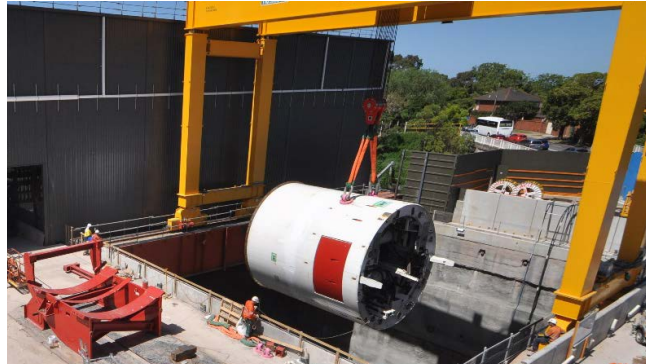
A TBM shield is lowered into the Chatswood dive by a 280-tonne gantry crane which was sustainably reused for TBM assembly across the project
