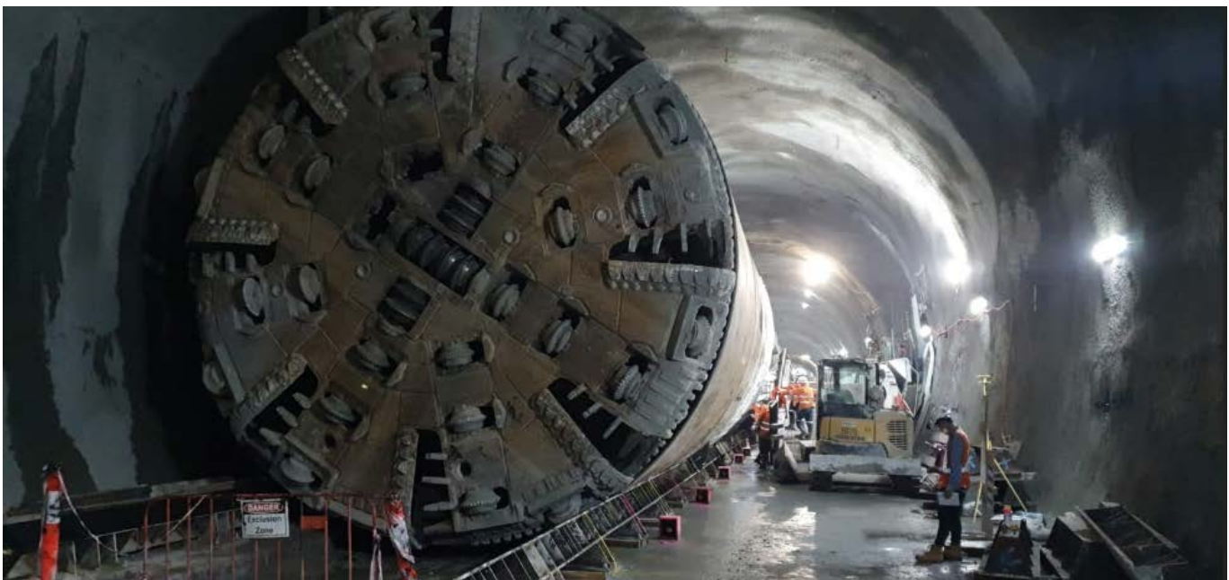
A protection slab was installed for the safe traverse of the TBM over the top of the Cross City Tunnel
