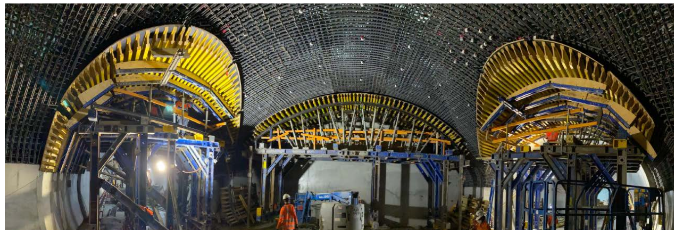
Complex cavern shapes and constrained working areas led to an innovative reinforcement solution
